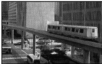
Courtesy of DTC/UTDC
